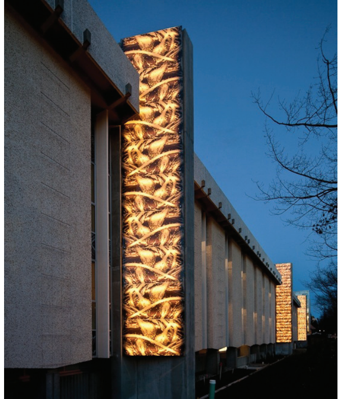
The glass concrete buttresses on the University of British Columbia biosciences building exterior feature digitally printed glass supplied by DSG Custom Glass and installed by John Peachy Associates.
