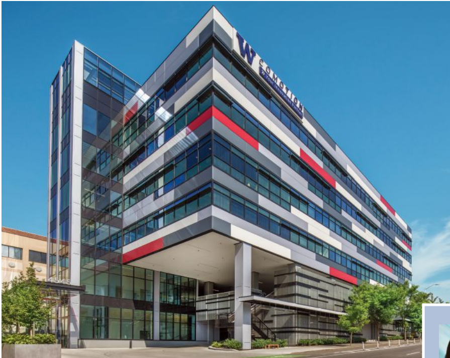
Another Seattle project, 4545 Roosevelt, uses a variety of bold colored metal cladding panels next to Vitro's Solarban 70XL, Solarban 67, Solarban 60 and Solarblue with ICD's Opaci-Coat-300 in Harmony Gray for the spandrel areas to create a checkerboard effect.
