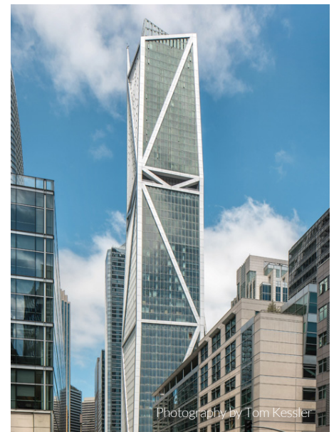
The angled design of 181 Fremont disrupts airflow to minimize wind load and reduce stress on the glass and frames.
